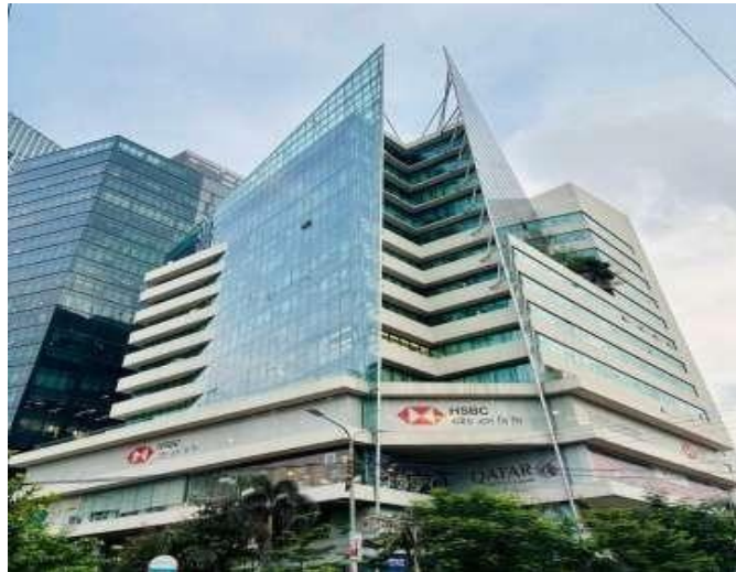
Figure 2: HSBC Management Office, Shanta Western Tower, Tejgaon
